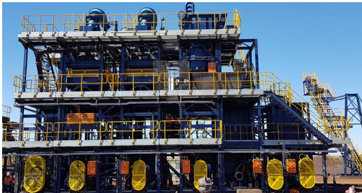
TRP being assembled on site – 11 th July 2019
