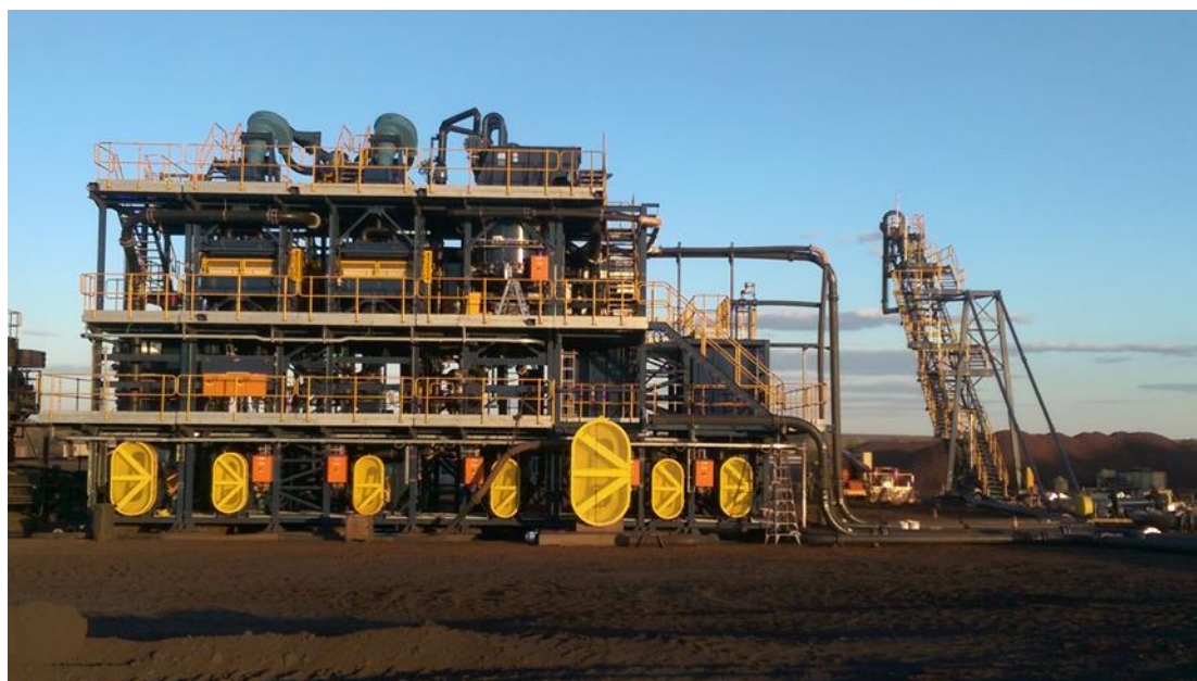
Completed construction of the TRP
